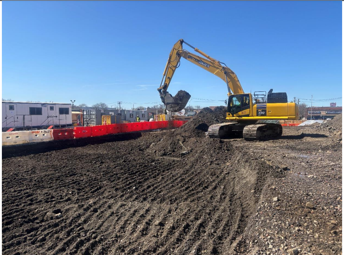
Photo 3 – United excavating in the western portion of the Site, facing north.
