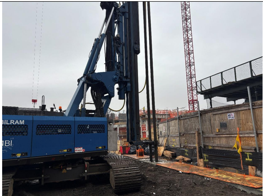
Photo 4 – RYC Turbos installing the soil mix wall along the southeastern boundary of the Site for the construction of the SOE, facing northeast.
