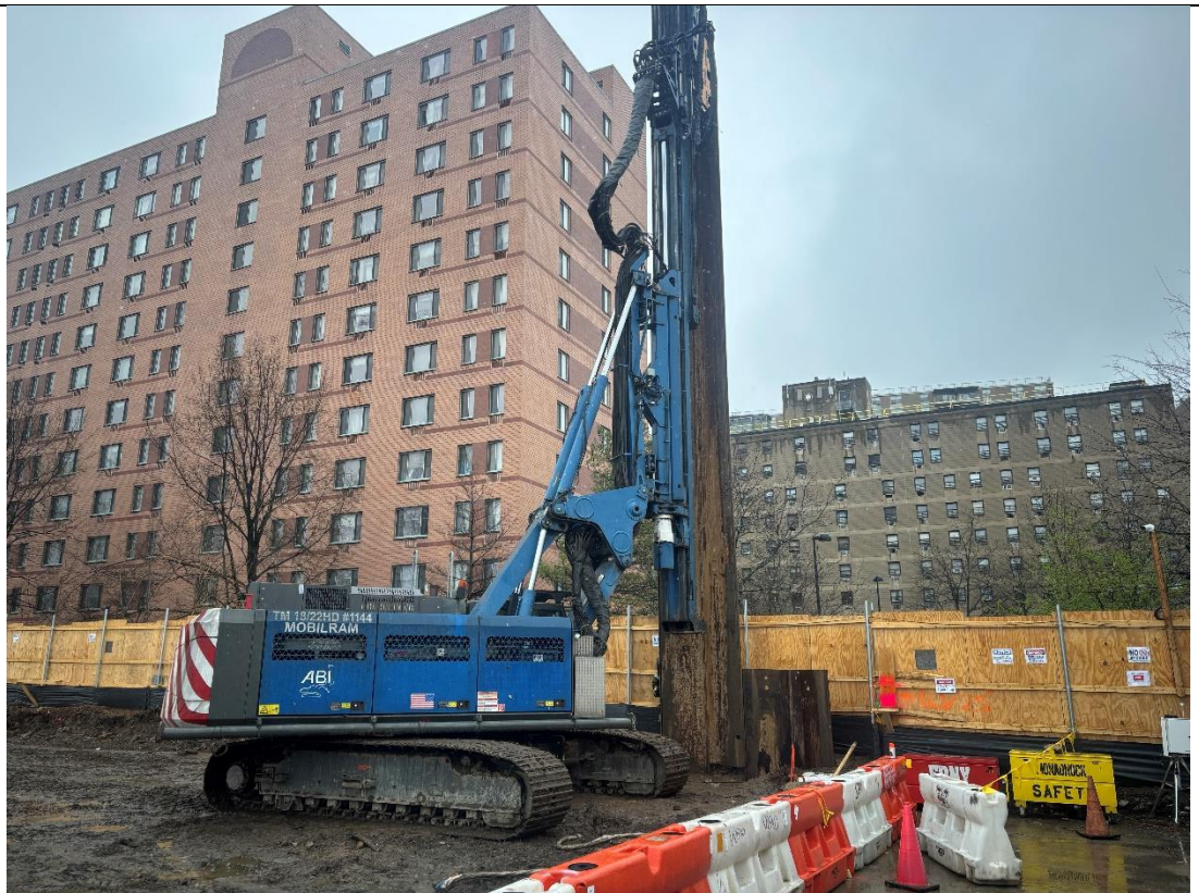
Photo 5 – RYC Turbos installing sheet piles in the southwestern portion of the Site, facing south.
