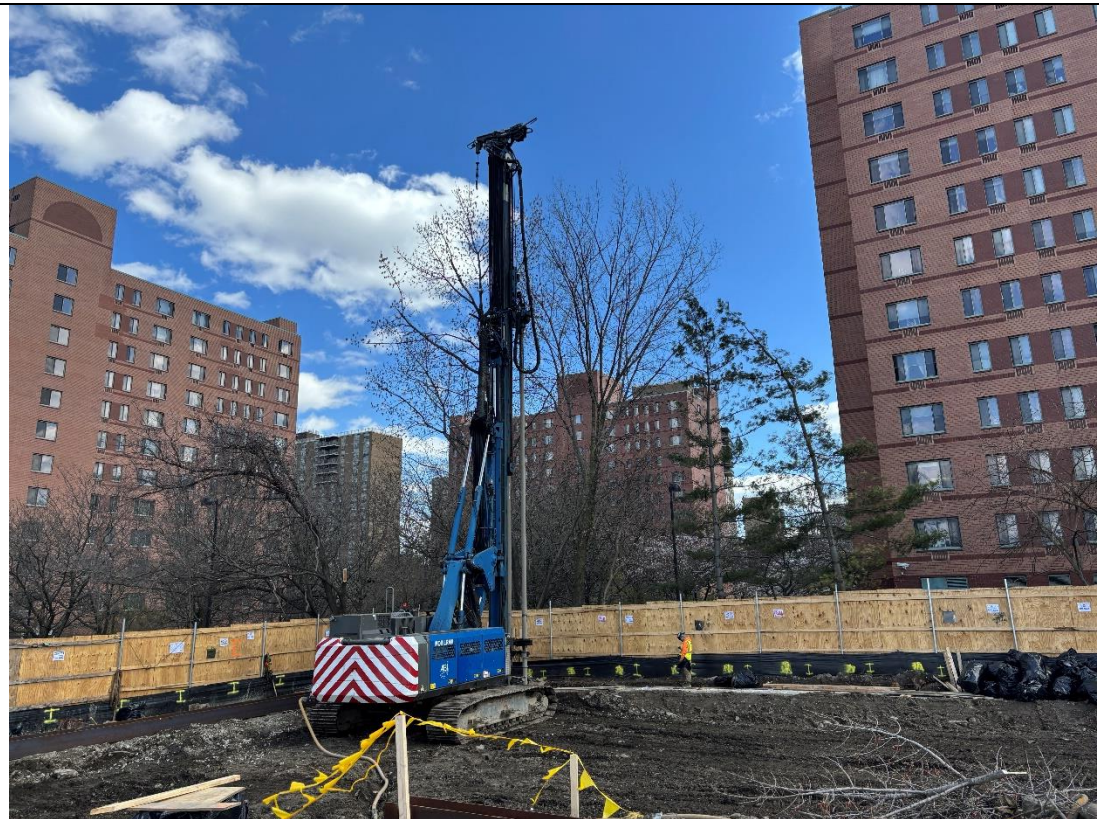
Photo 4 – RYC Turbos installing the soil mix wall along the southeastern boundary of the Site, facing southeast.
