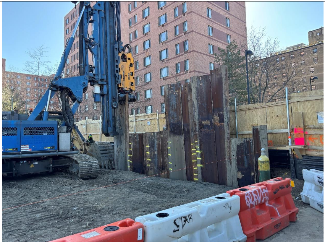
Photo 4 – RYC Turbos installing sheet piles along the southwestern boundary of the Site, facing southeast.
