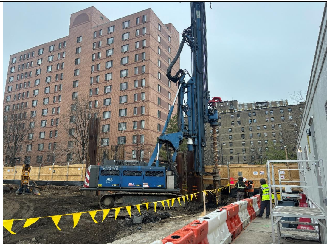
Photo 4 – RYC Turbos drilling in the southwestern portion of the Site to facilitate sheet pile installation, facing south.
