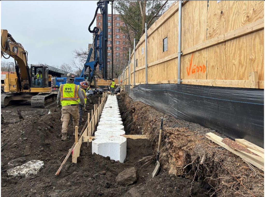
Photo 3 – RYC Turbos installing the SOE guide wall in the southern portion of the Site, facing east.
