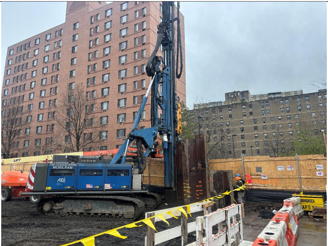
Photo 3 – RYC Turbos removing sheet piles in the southwestern portion of the Site, facing south.
