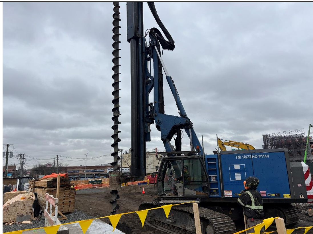
Photo 4 – RYC Turbos drilling in the western portion of the Site to facilitate sheet pile installation, facing north.
