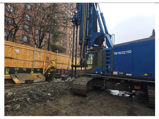
Photo 2 – RYC Turbos installing the soil mix wall in the southern portion of the Site, facing east.
