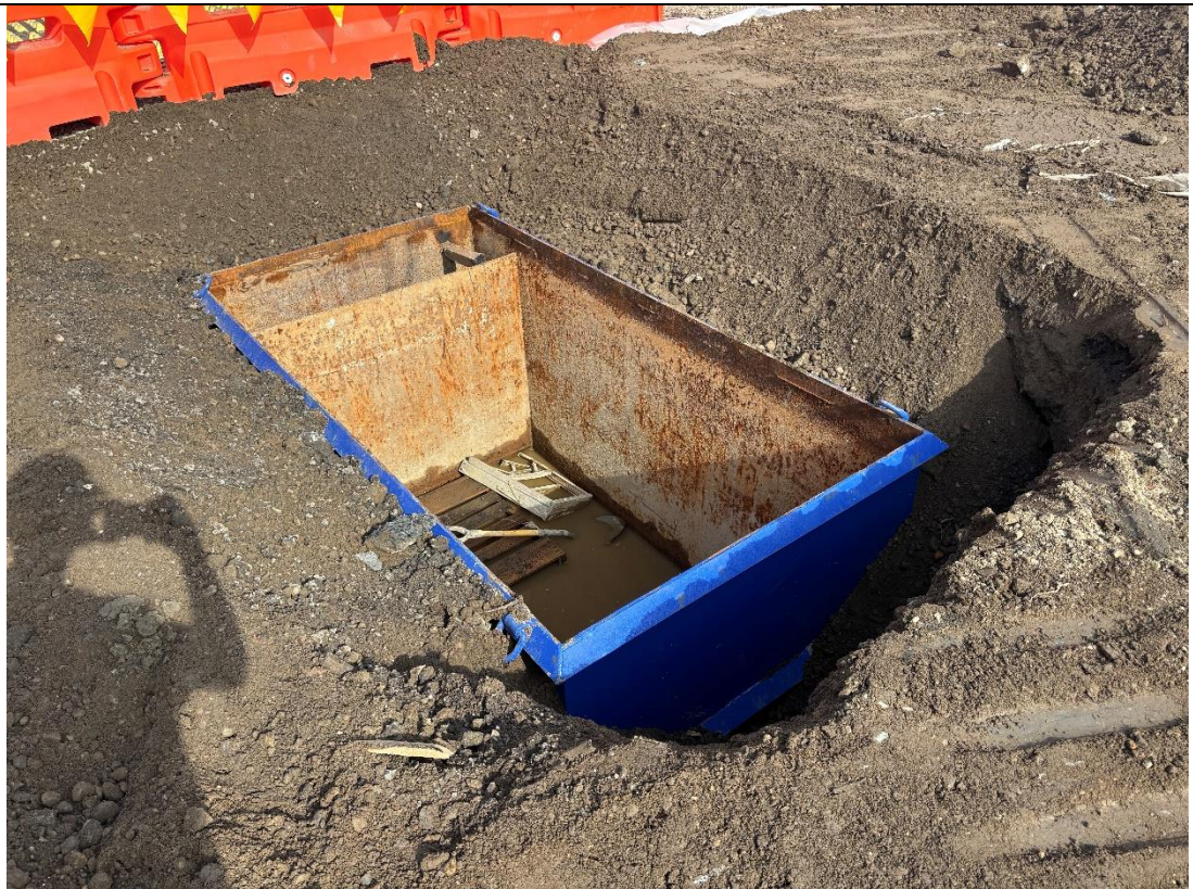
Photo 6 – View of the truck wash water collection and settling tank placed within the excavated area in the northern portion of Lot 100, facing southeast.
