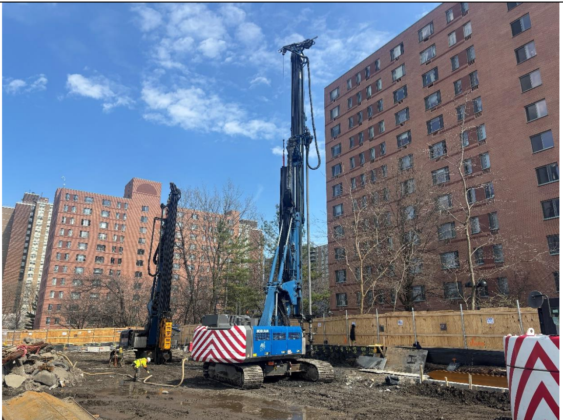
Photo 4 – RYC Turbos installing the soil mix wall in the southern portion of the Site, facing southeast.
