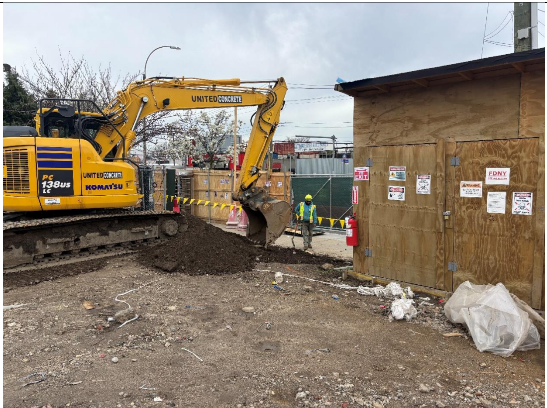
Photo 5 – United excavating in the northern portion of Lot 100 for the construction of a truck wash station, facing northwest.
