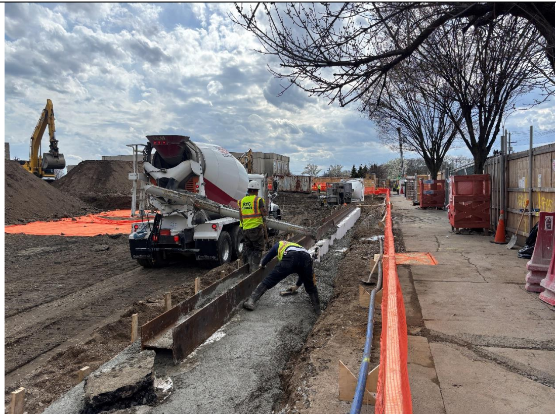
Photo 4 – RYC Turbos installing the soil mix guide wall in the northern portion of the Site, facing west.
