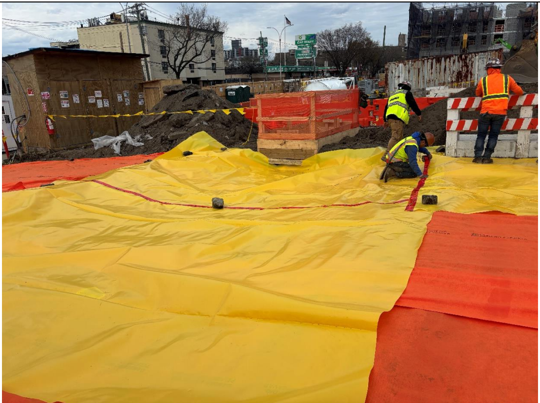
Photo 6 – United installing Stego wrap above the excavated area in the northern portion of Lot 100 for the construction of the truck wash station, facing east.
