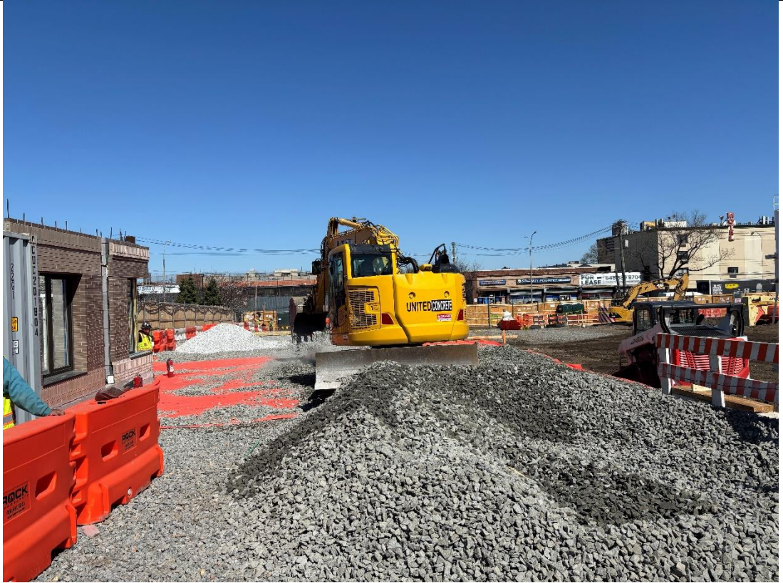
Photo 3 – United placing the imported 1.5-inch clean stone on Lot 100 for the construction of the logistical zone, facing north.
