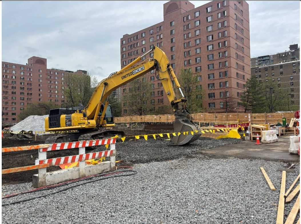
Photo 3 – United placing 1.5-inch stone above the truck wash station in the western portion of the Site, facing southeast.
