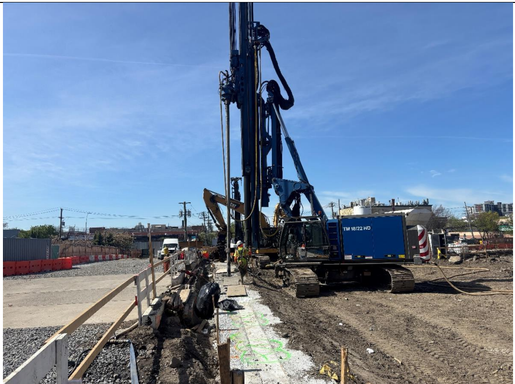
Photo 4 – RYC Turbos installing the soil mix wall along the western boundary of the Site, facing north.
