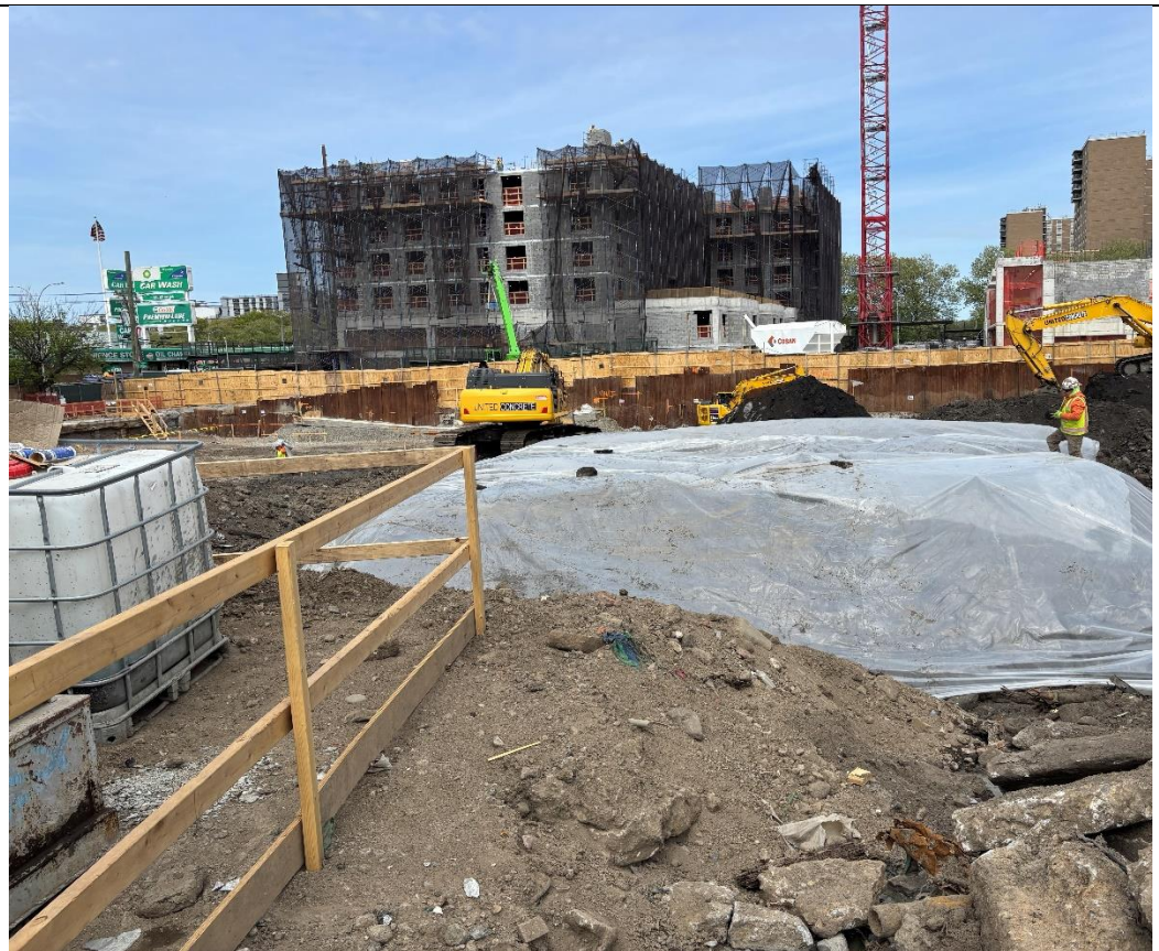
Photo 4 – Stockpile ST-31 being covered with polyethylene sheeting at the end of the day, facing east.
