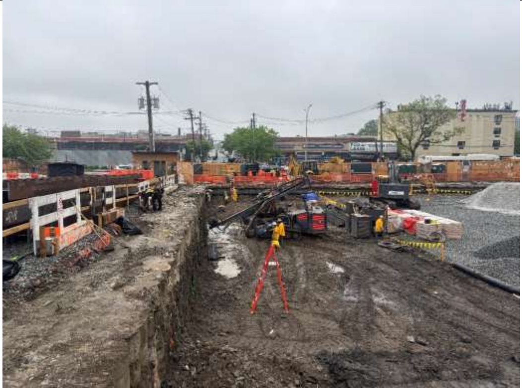
Photo 3 – RYC Turbos installing tiebacks in the northwestern portion of the Site, facing north.
