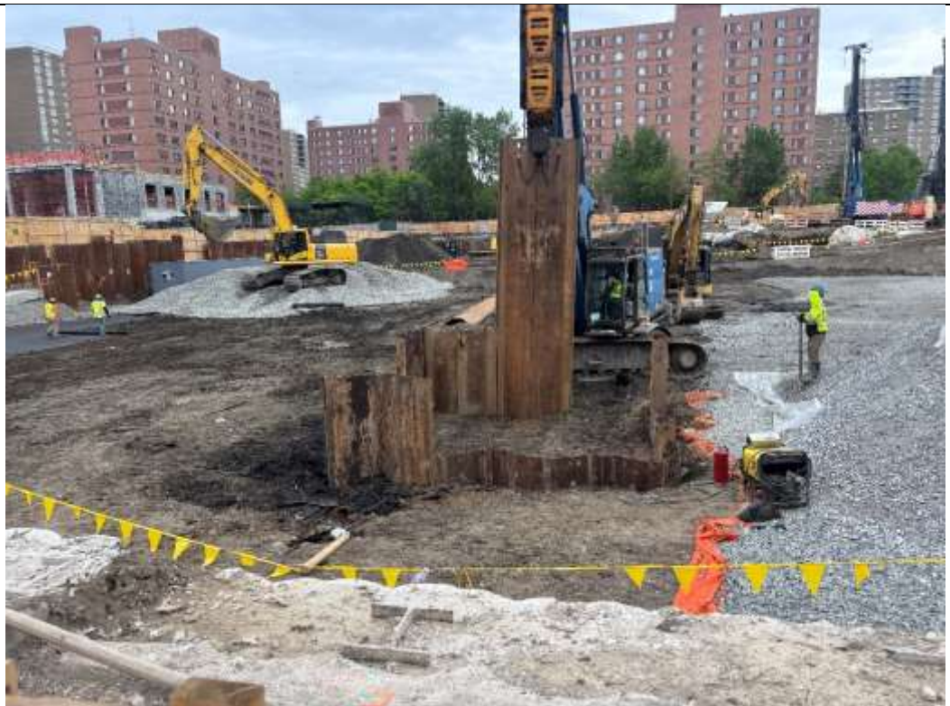
Photo 4 – RYC Turbos installing sheet piles in the northeastern portion of the Site, facing south.
