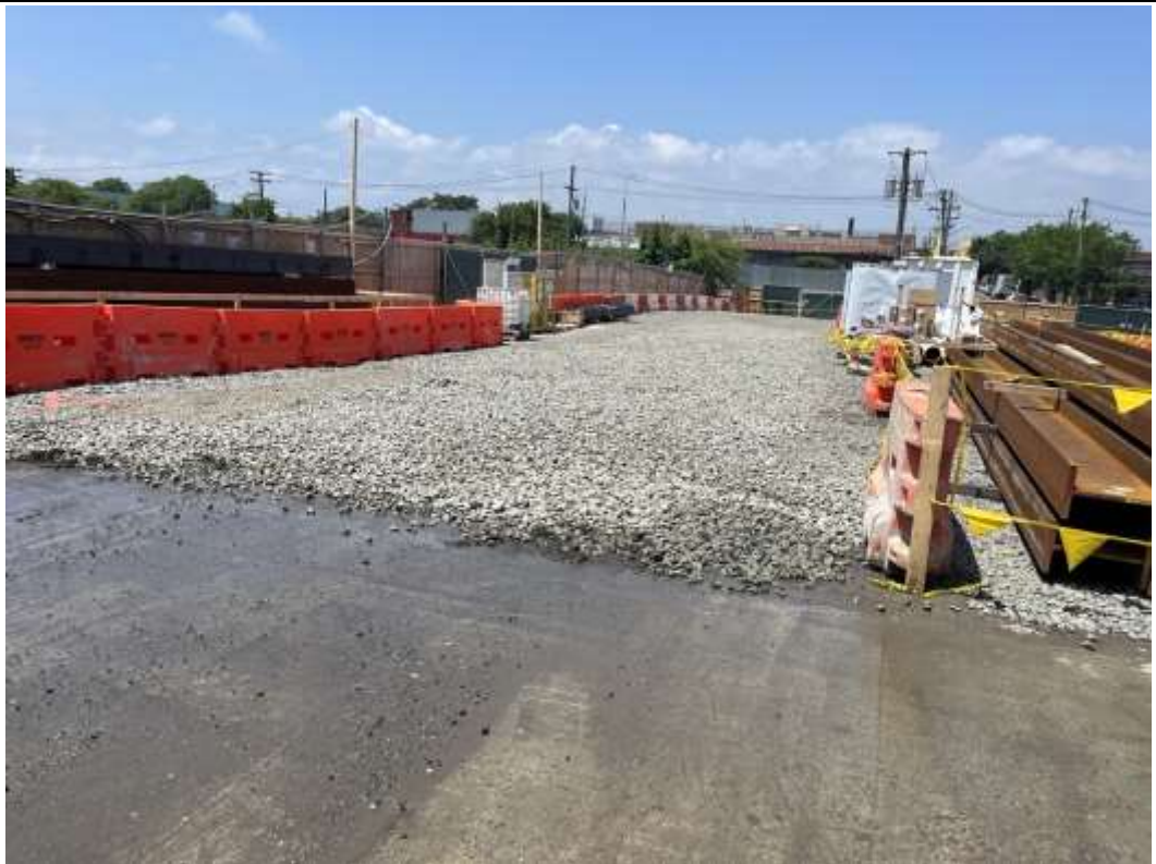
Photo 4 – View of imported 1.5-inch stone spread on Lot 100, facing north.
