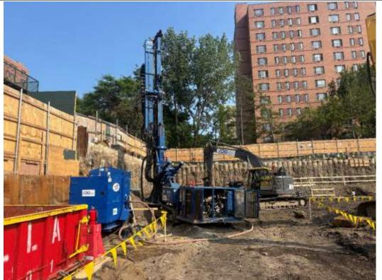
Photo 4 – Morris-Shea installing foundation piles in the central portion of the Site, facing south.
