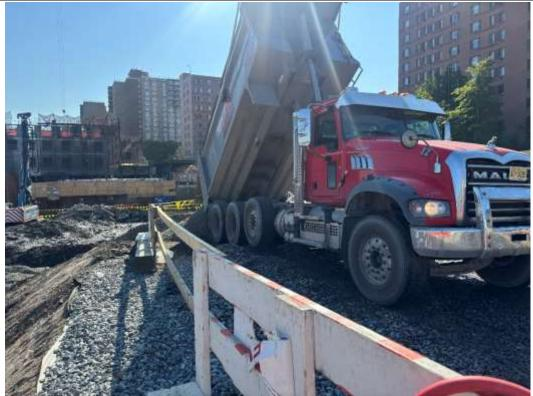
Photo 2 – View of the previously excavated area in the central portion of the Site for the removal of obstructions backfilled with imported 1.5-inch clean stone, facing southwest.
