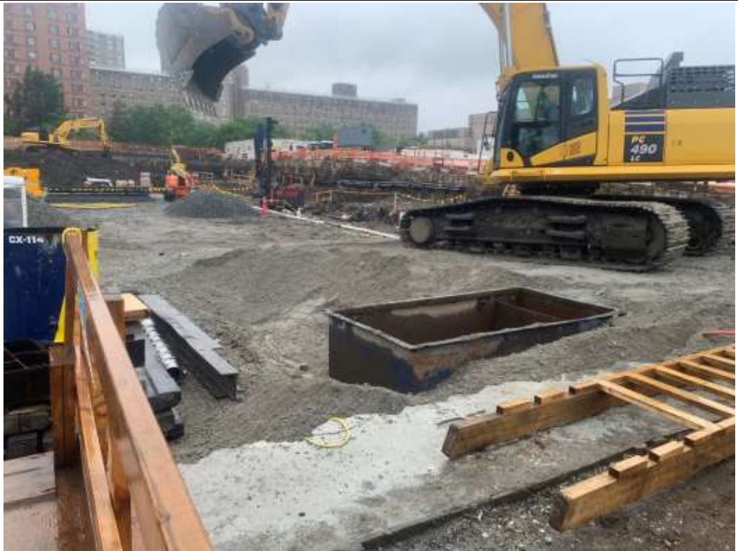
Photo 3 – United placing the settling tank east of truck ramp TR-4, facing southwest.
