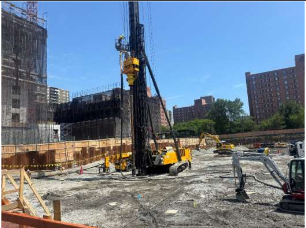
Photo 4 – Morris-Shea installing deep foundation piles in the northeastern portion of the Site, facing southeast.
