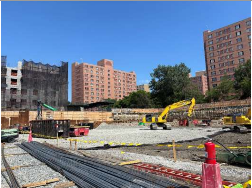
Photo 4 – Imported clean 1.5-inch stone placed above Mirafi filter fabric in the eastern portion of the Site, facing southeast.
