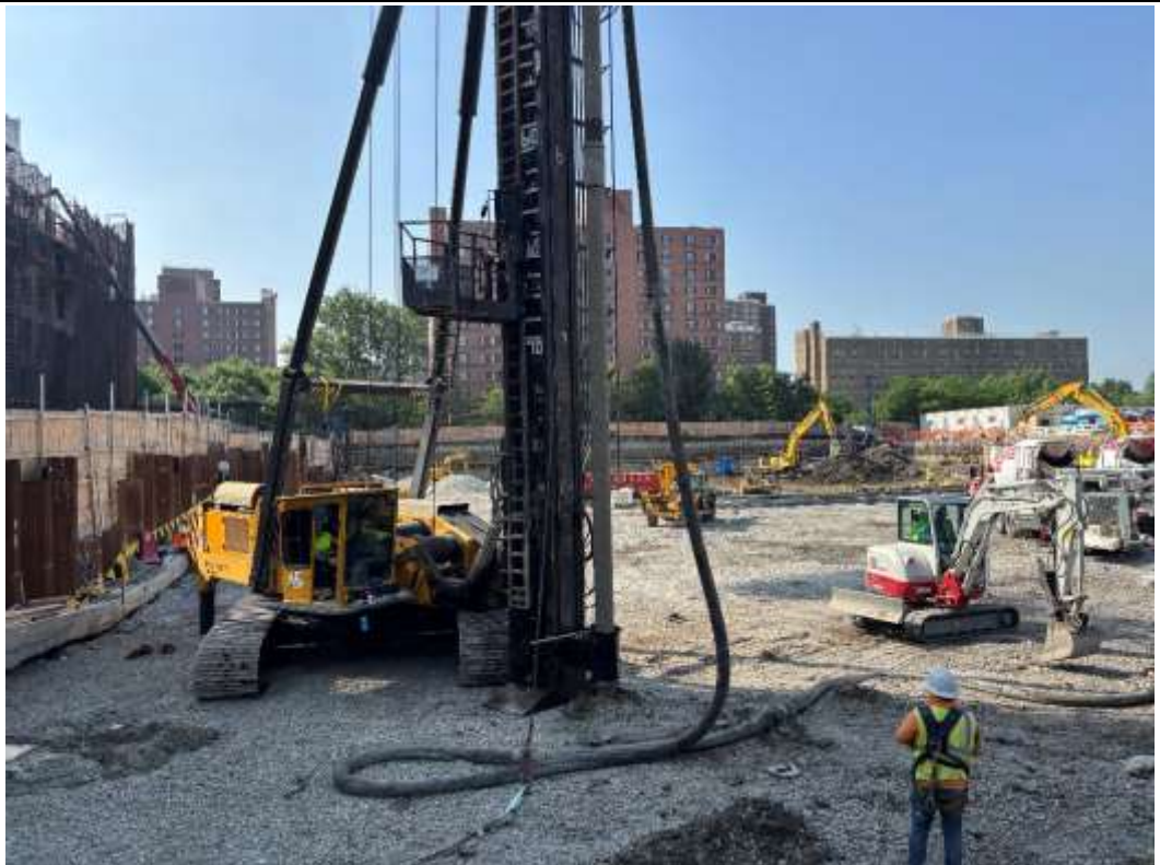
Photo 4 – Morris-Shea installing deep foundation piles in the northeastern portion of the Site, facing south.
