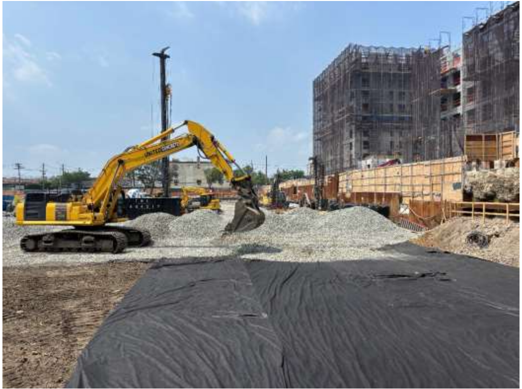
Photo 3 – United placing previously imported 1.5-inch clean stone from stockpile ST-62 in the southeastern portion of the Site, facing north.
