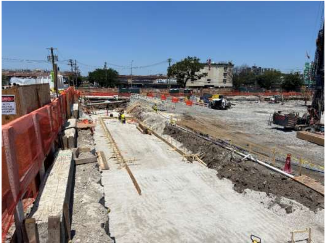
Photo 3 – United installing formwork in the northwestern portion of the Site for the construction of the detention tank foundation, facing north.
