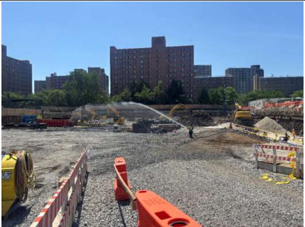
Photo 4 – United spraying water as a preventative dust control measure, facing south.
