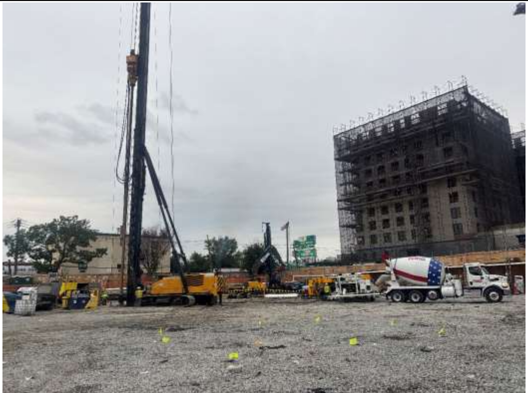
Photo 4 – Morris-Shea installing deep foundation piles in the northern portion of the Site, facing northeast.
