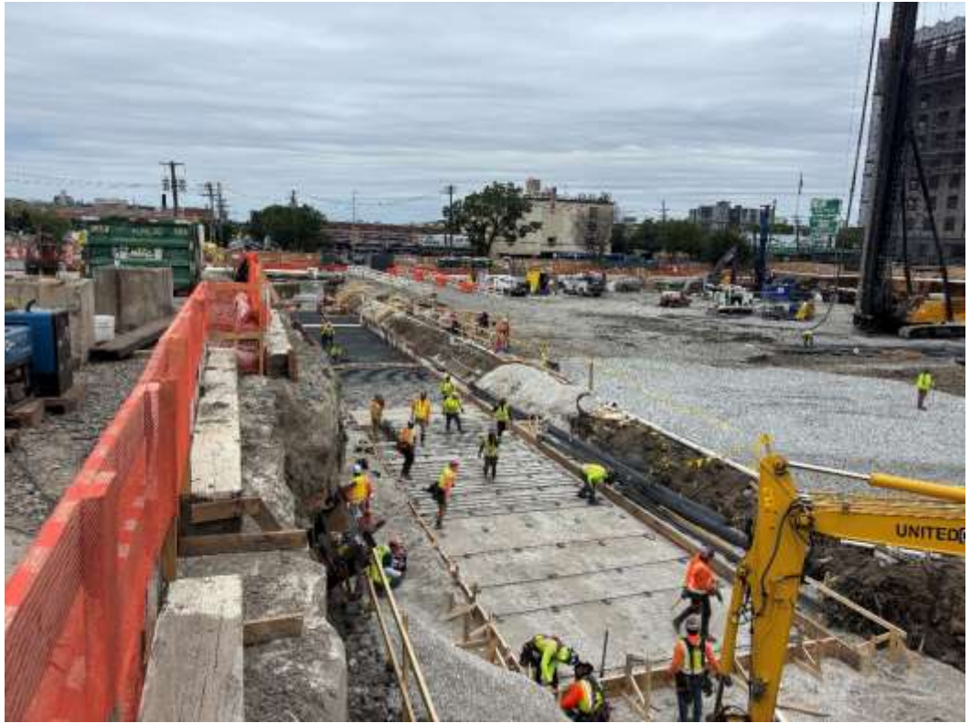
Photo 3 – United installing rebar and formwork for the construction of the detention tank foundation in the western portion of the Site, facing north.
