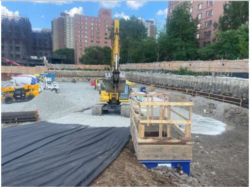
Photo 3 – View of United placing DGA on top of truck ramp TR-5 within the southwestern portion of the Site, facing west.
