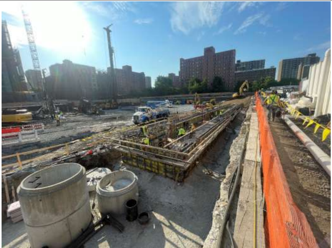
Photo 1 – United installing rebar and formwork for the construction of the detention tank foundation, facing south
