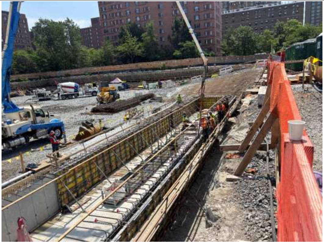
Photo 3 – United pouring concrete for the construction of the detention tank walls, facing south.
