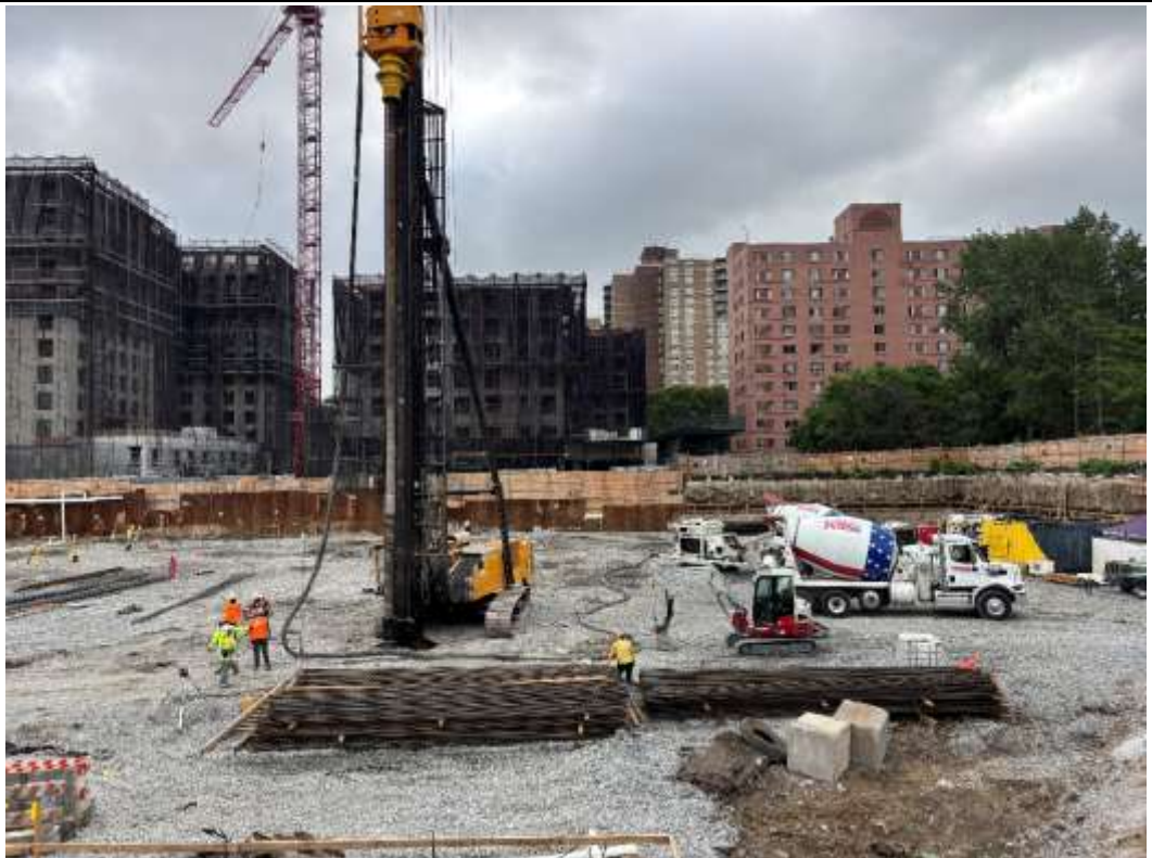
Photo 4 – Morris-Shea installing deep foundation piles in the central portion of the Site.
