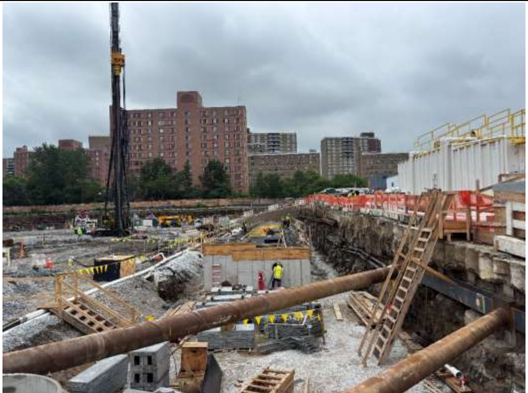
Photo 4 – United installing rebar and formwork for the construction of the detention tank, facing south.
