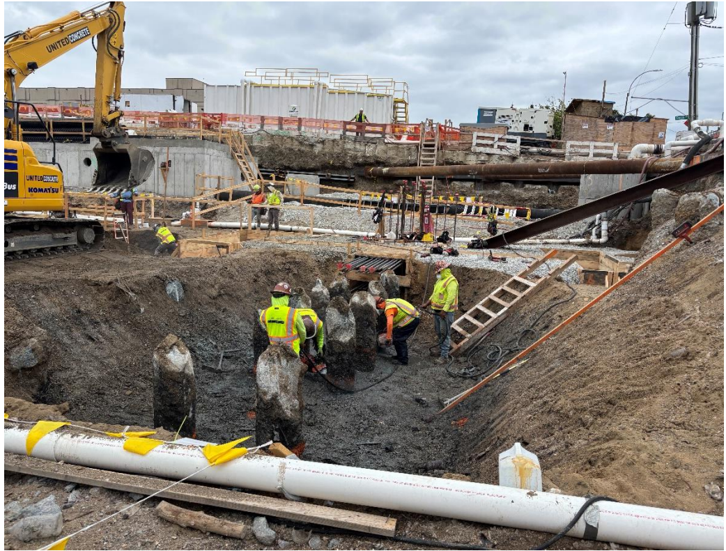
Photo 3 – United cutting piles to grade in the northern portion of the Site, facing west.
