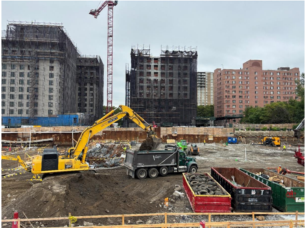
Photo 1 – United loading material for off-Site disposal to Clean Earth Carteret, facing east.
