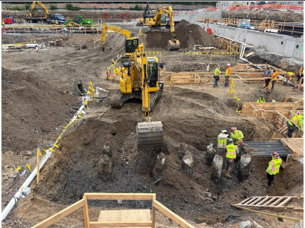
Photo 2 – United excavating in the northern portion of the Site, facing south.
