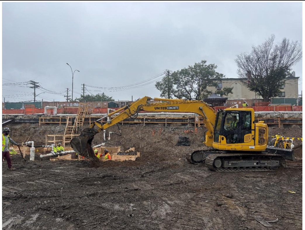
Photo 4 – United backfilling around pile cap formwork with clean fill, facing north.
