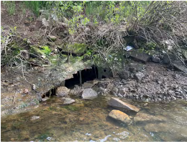
Photograph 1: Stormwater outfall, as seen from Coney Island Creek; view facing north.
