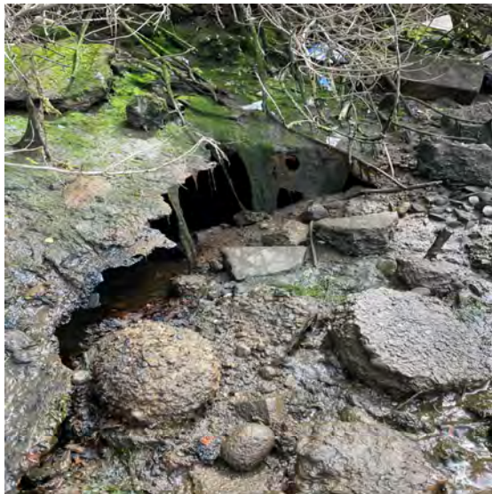
Photograph 3: Close-up view of outfall.
