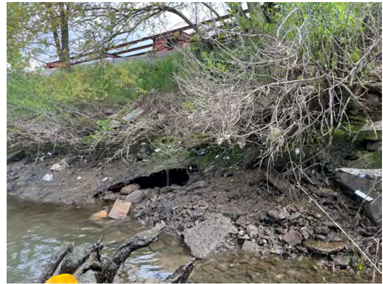
Photograph 2: Stormwater outfall; view facing northwest.
