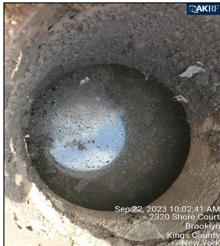
Photograph 3: Interior of catch basin prior to cleaning.
