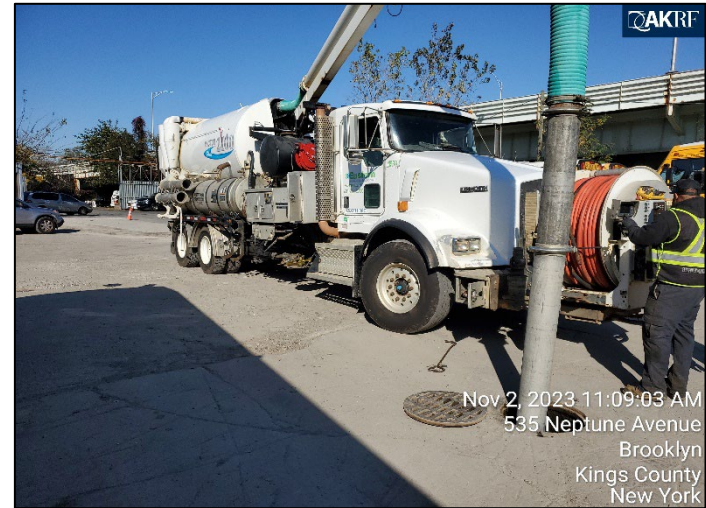
Photograph 6: High-powered vacuum truck (guzzler) removing accumulated sediment from catch basin.
