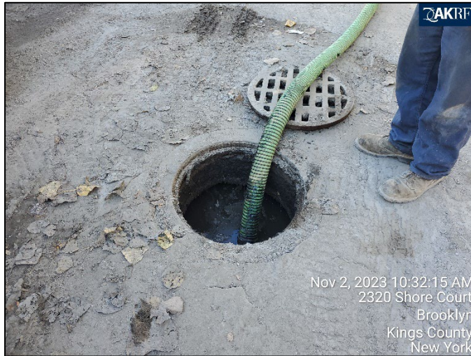
Photograph 5: Removal of standing liquids from catch basin prior to sediment removal.
