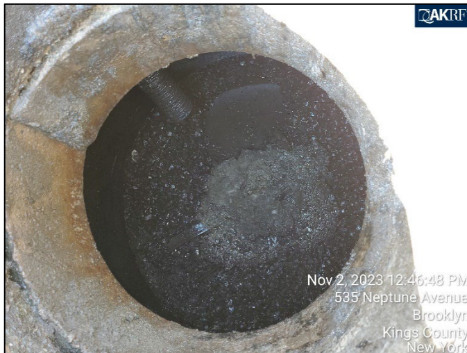
Photograph 7: Interior view of catch basin CB-02 after cleaning, with concrete and asphalt at the bottom.
