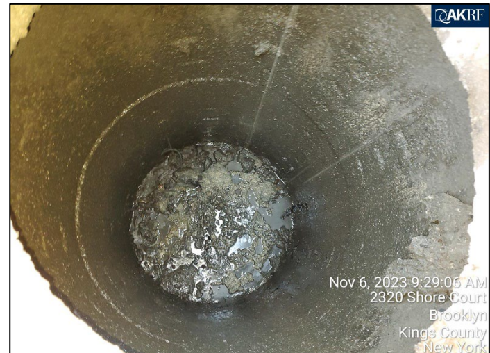
Photograph 8: Interior view of catch basin CB-05 after cleaning, with concrete and rebar at the bottom.
