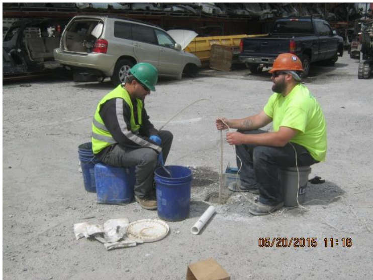
Photograph 3. Well development activities at groundwater monitoring well MW-3.
