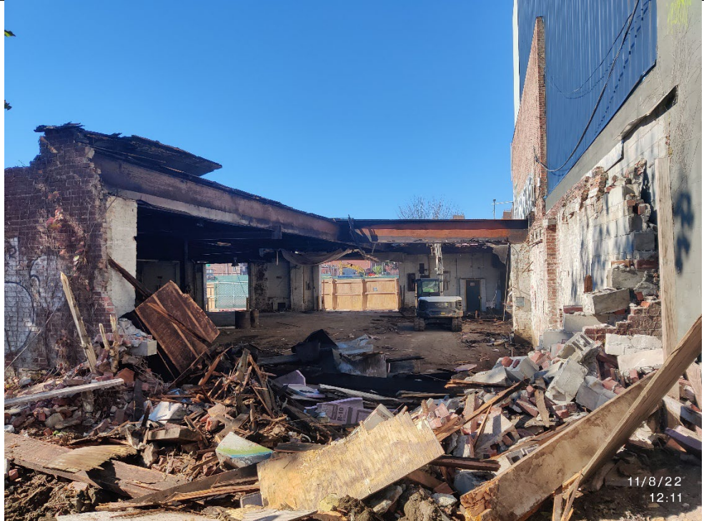
Photo 3 – Representative view of building demolition in progress within large warehouse structure located on the western portion of the Site.
