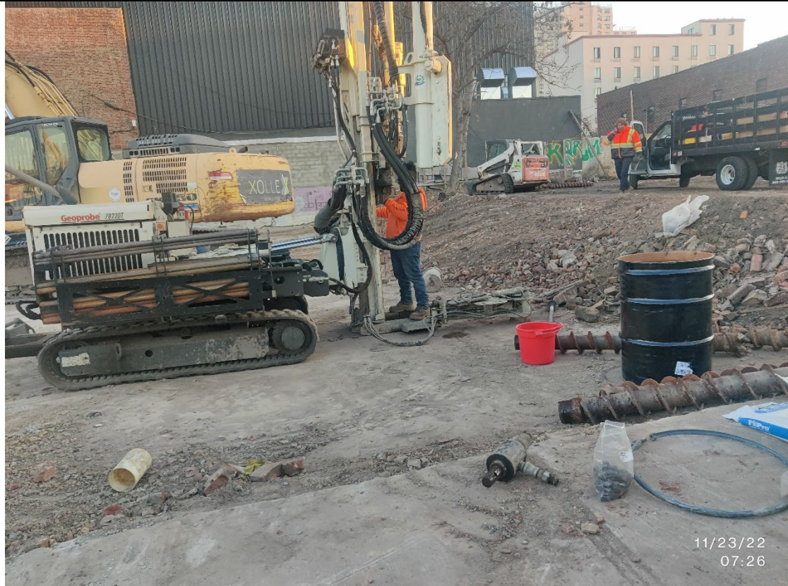
Photo 1 – Installation of shallow GW-8 well begins.
