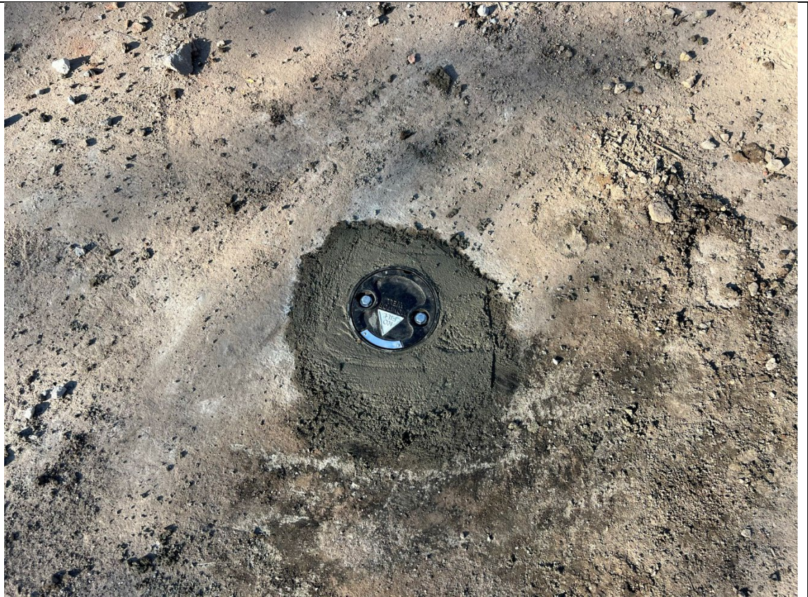
Photo 2 – Photo of shallow GW-6 well Completed.
