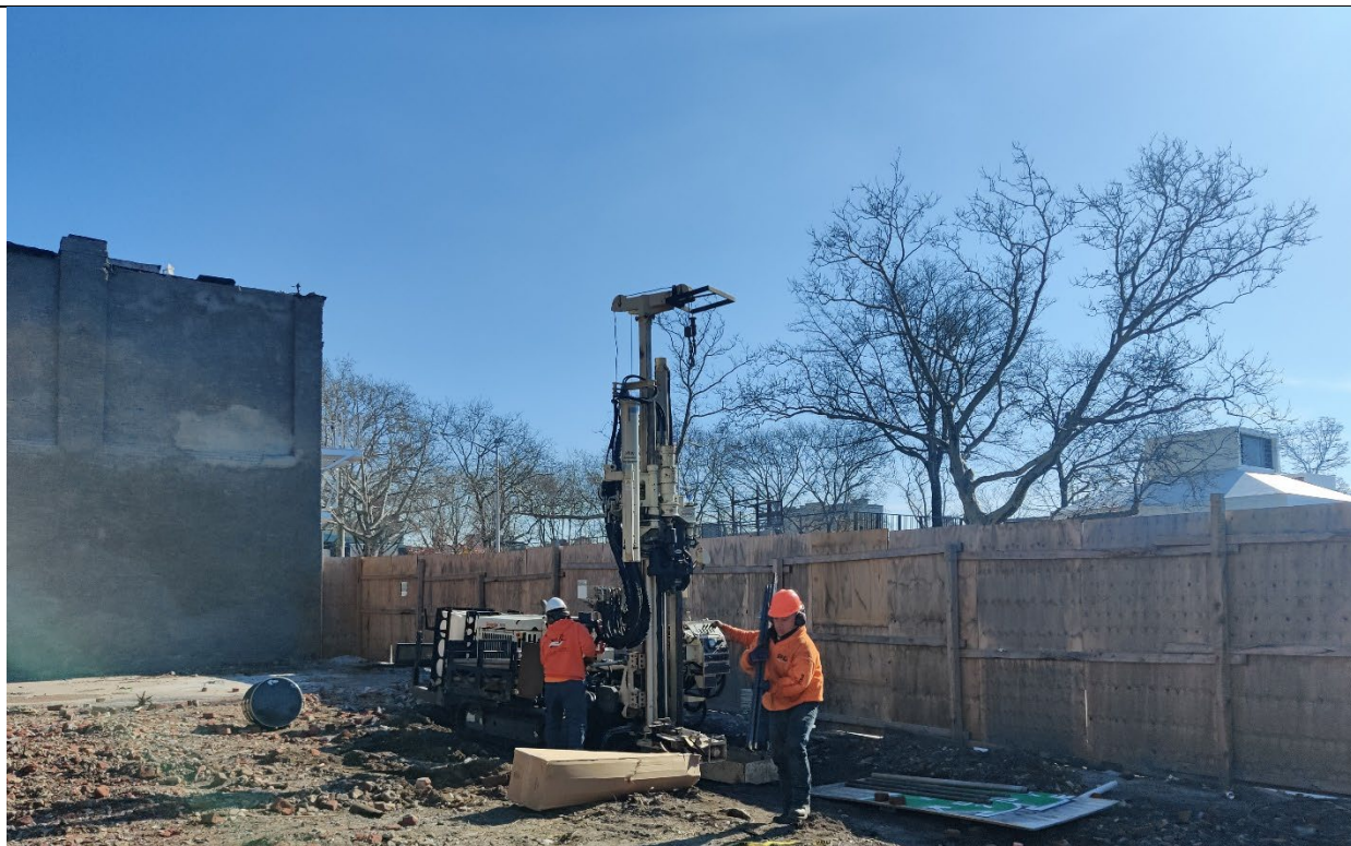
Photo 3- Representative photo of drilling activities commencing at DB-1.
