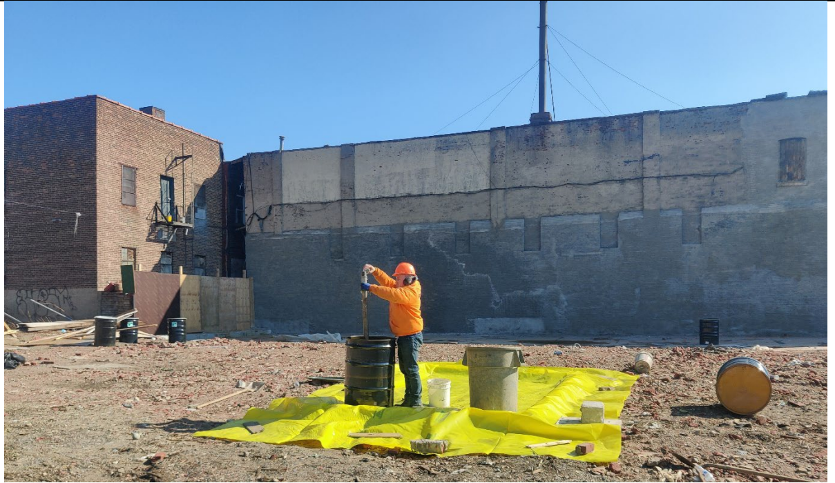
Photo 2 – Representative view of decon basin in use.
