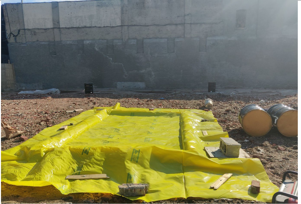
Photo 1 – Representative photo of decon basin
