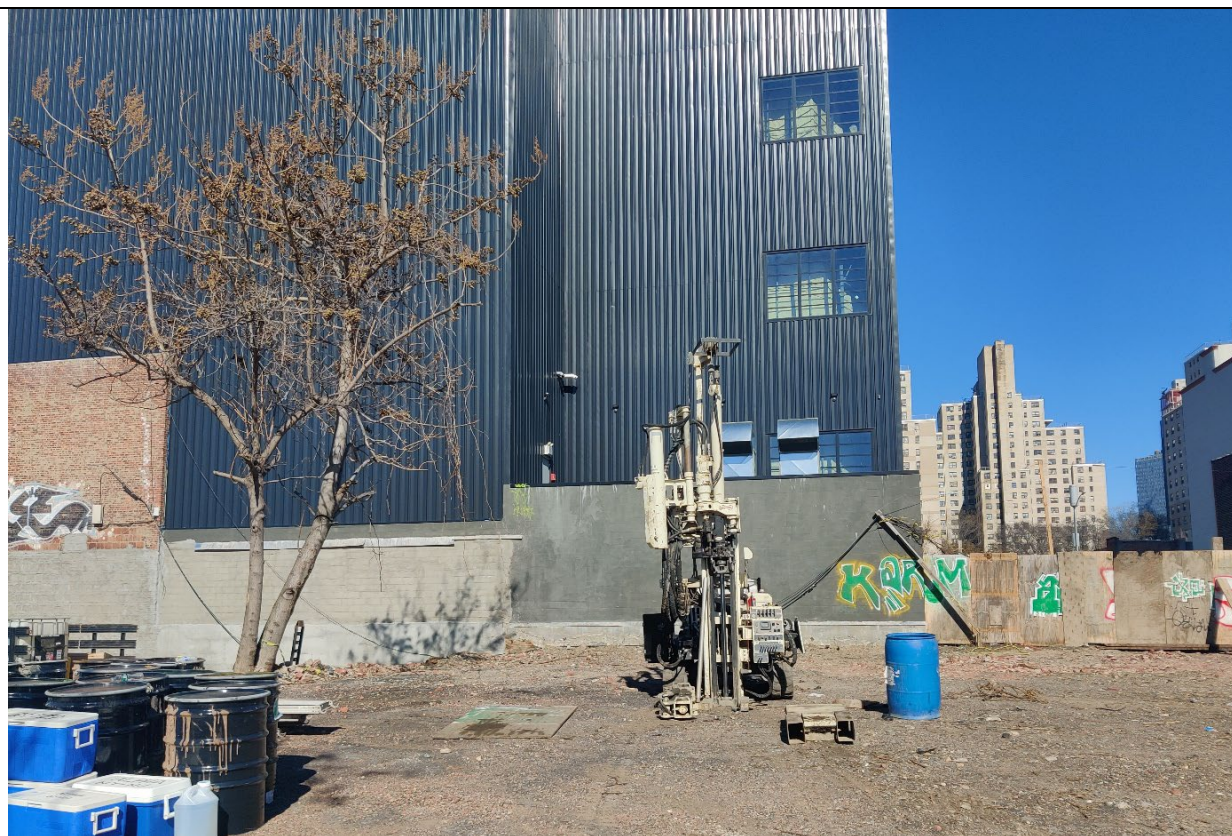
Photo 4- DB-5 Drilling location
