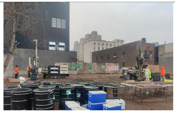
Photo 2-Representative photo of boring DB-19 with intervals from grade to 40' bgs. This boring location was impacted with MGP Coal Tar beginning at 3' bgs.
