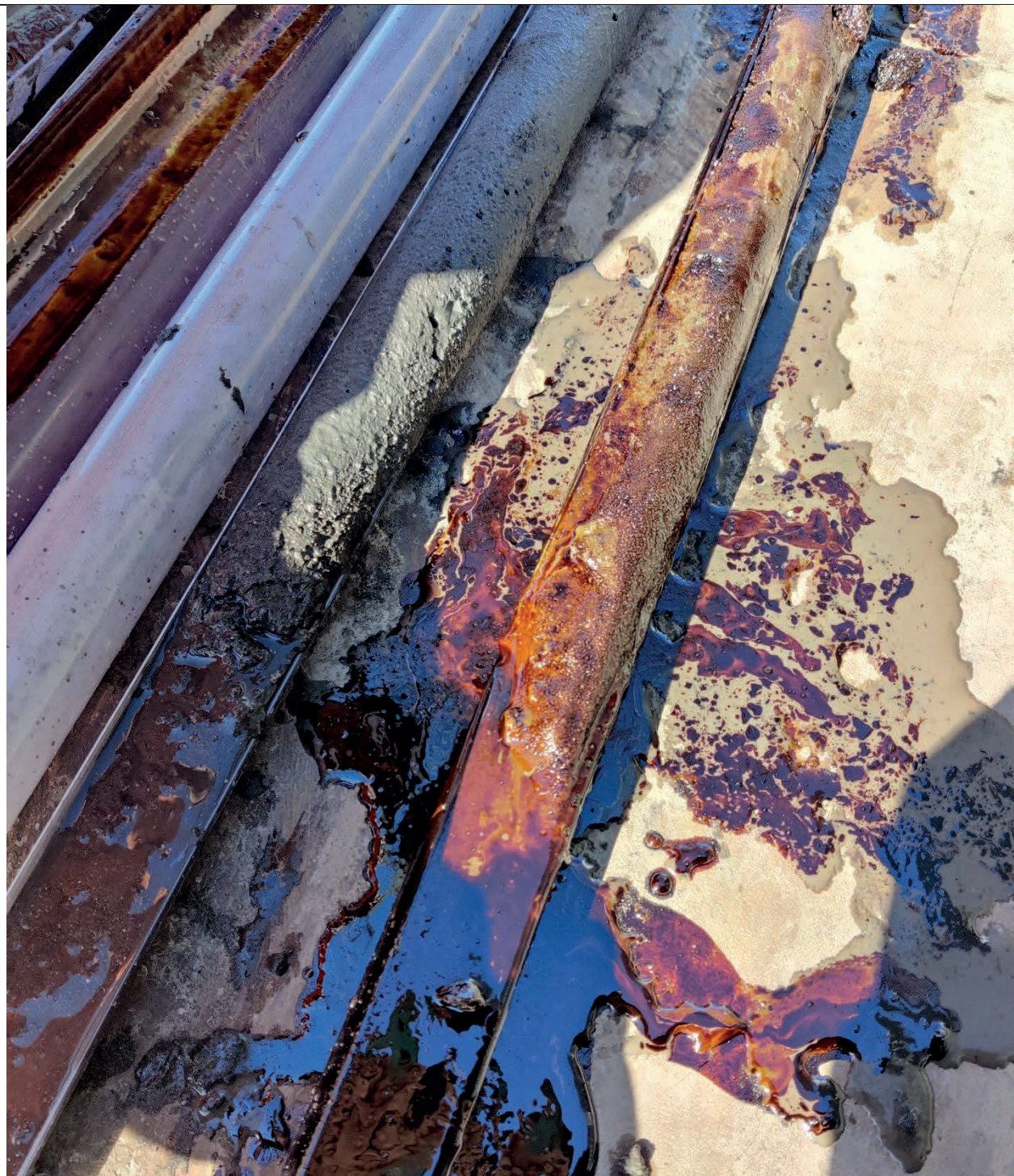
Photo 2- Representative view of boring DB-11, impacted with MGP coal tar at the 30-35' interval.
