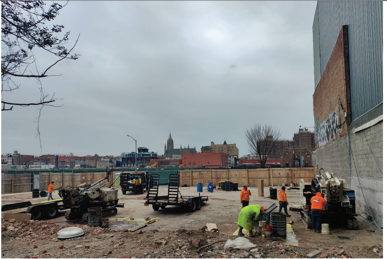
Photo 1- Representative view of the Site at the start of the days activities.
