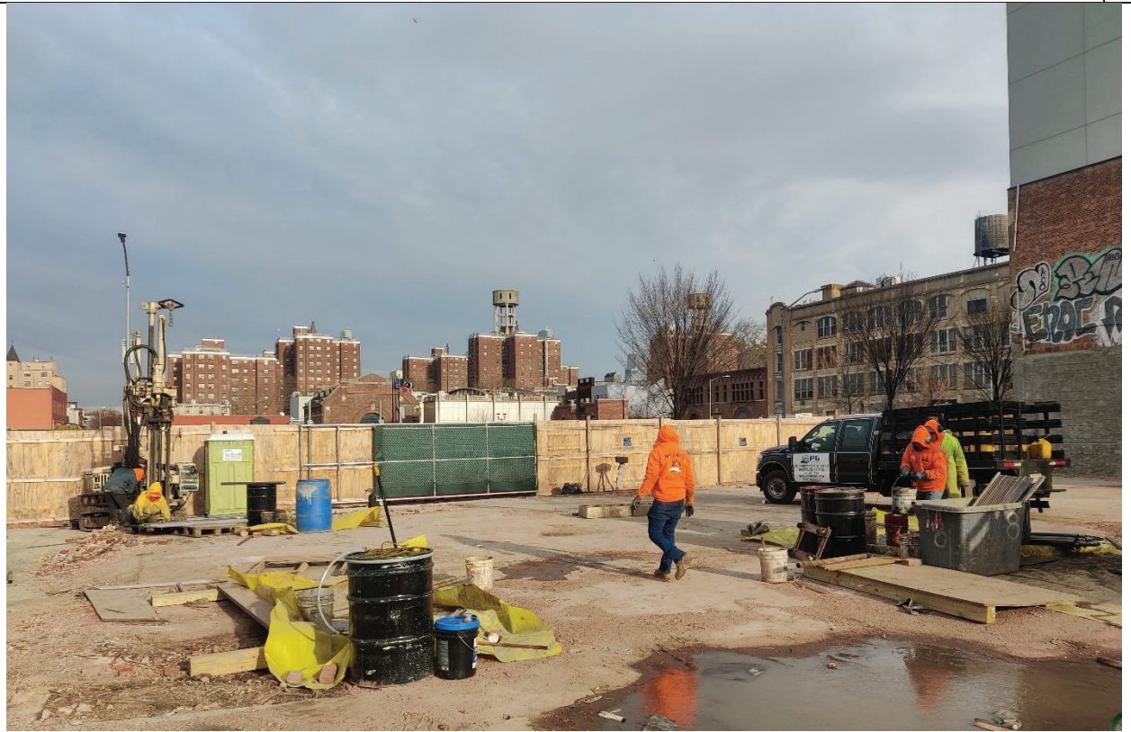
Photo 1- Representative view of the Site at the start of the days activities.
