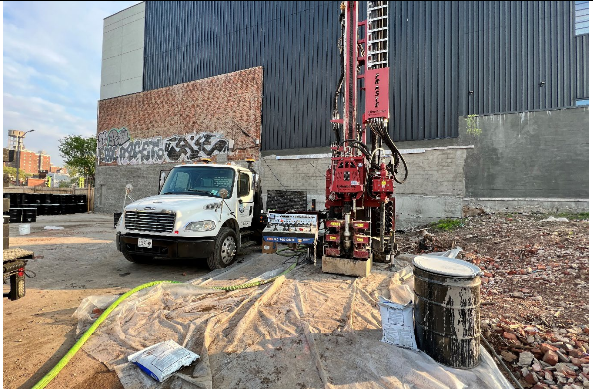
Photo 1 – Representative view of site at beginning of workday.
