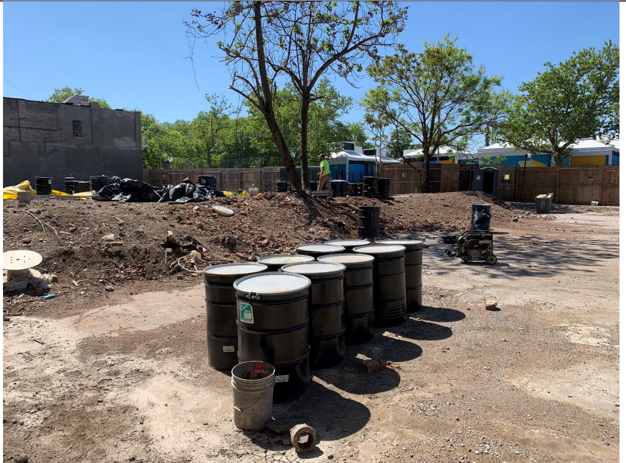
Photo 1 – Representative view of Site with empty drums staged near CW- 4 for MW purging.
