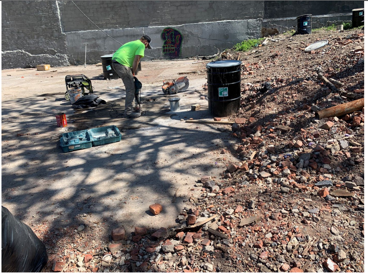
Photo 2 – Representative view of manhole covers placement in CW-4.
