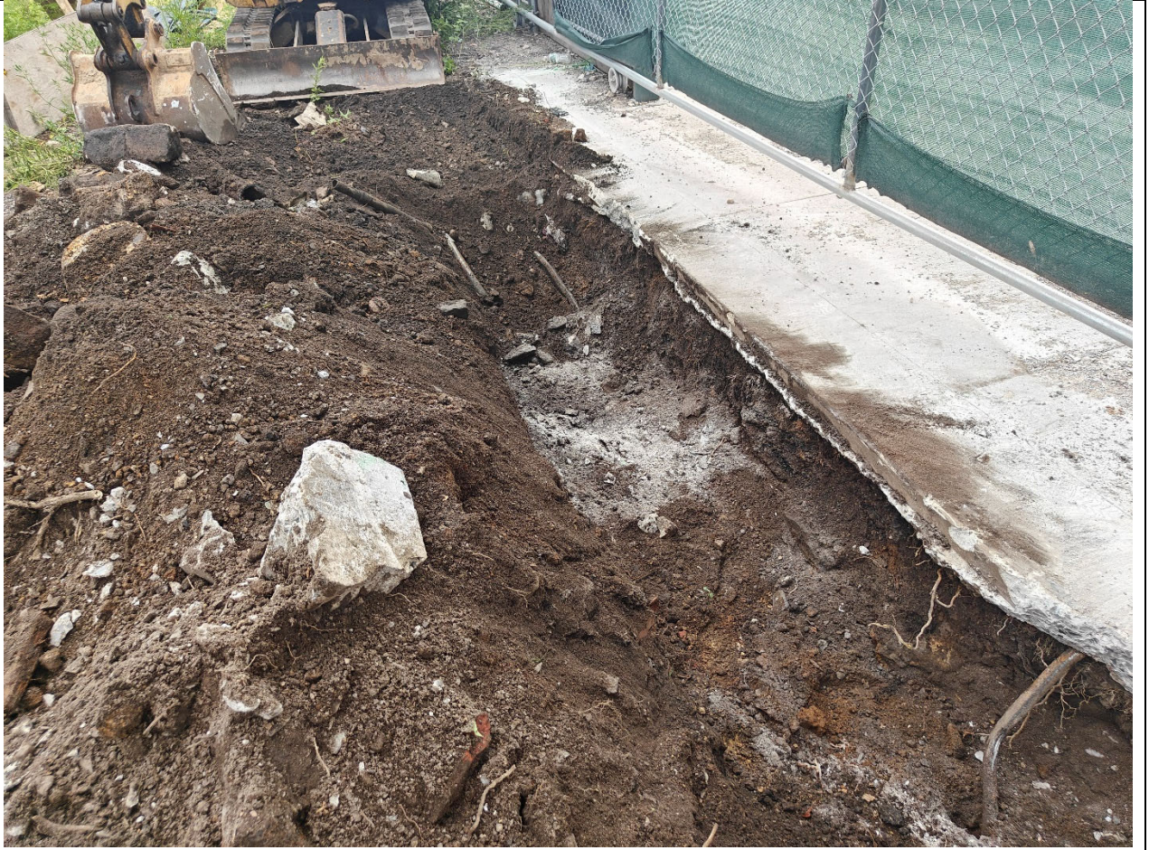
Photo 2- Representative photo of trenching
