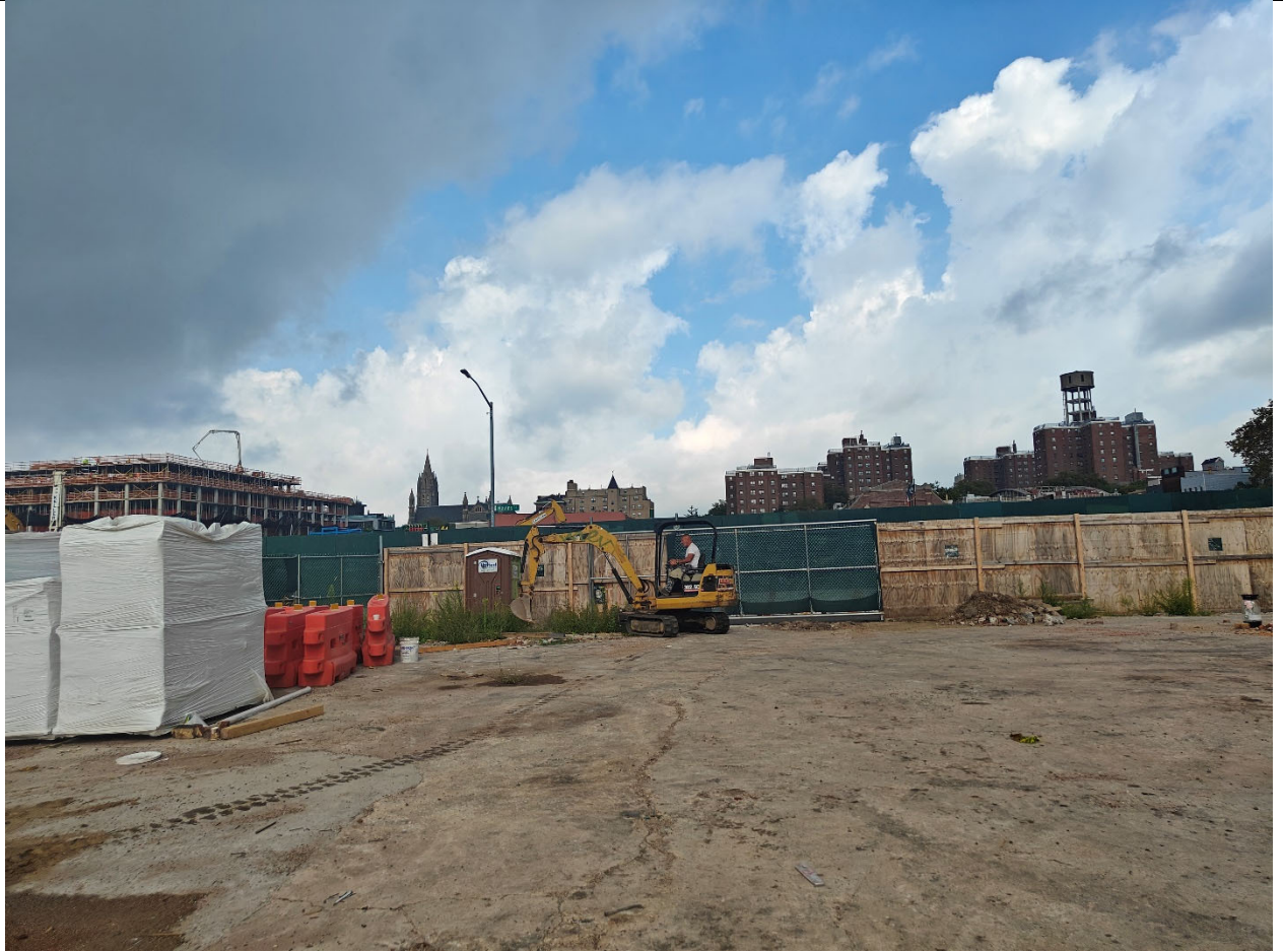
Photo 1- Site at the beginning of trenching activities
