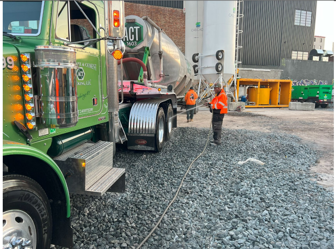
Photo 3- Representative photo of tires being washed.
