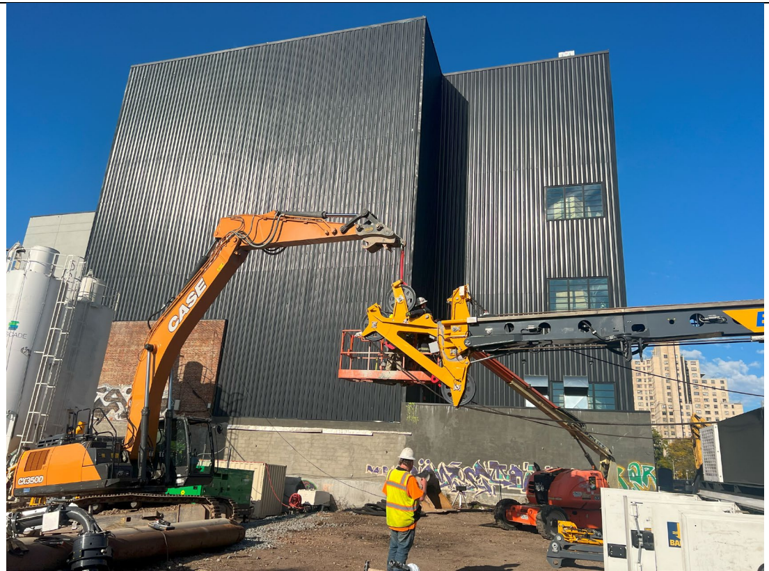
Photo 2- Representative photo of work being done on the rig.
