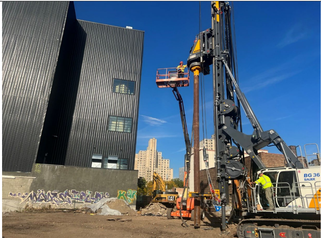
Photo 2- Representative photo of Cascade working on the rig.
