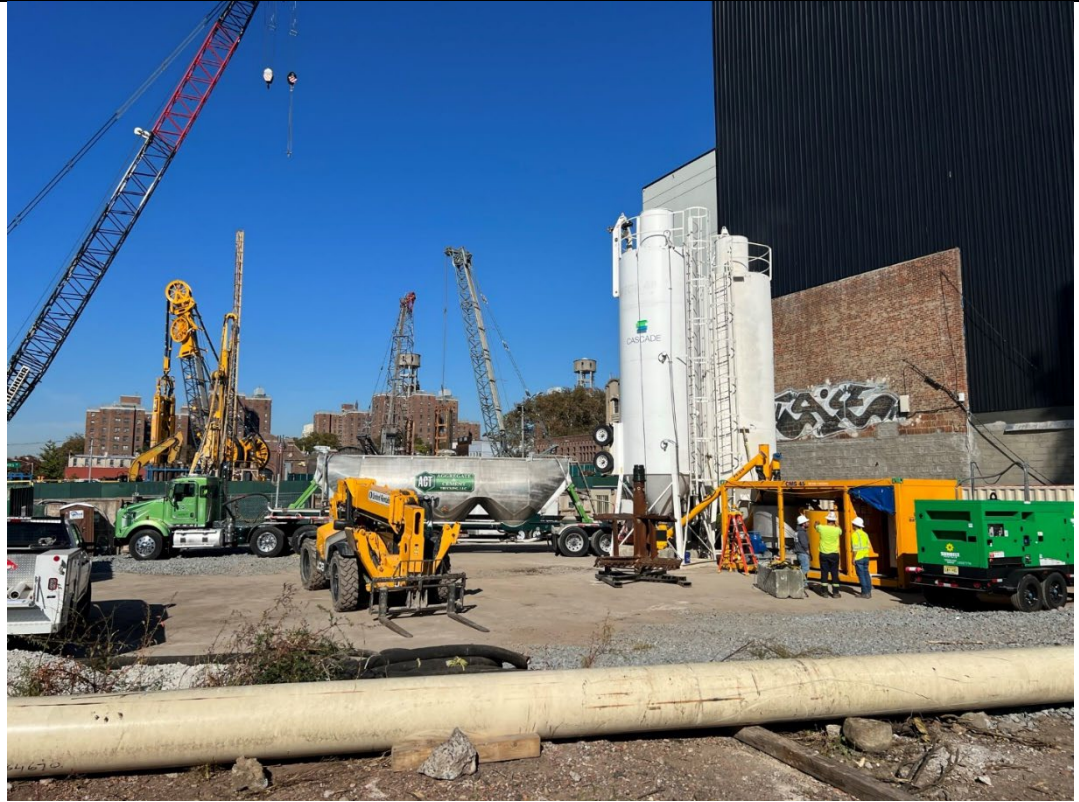
Photo 1- Representative photo of Cascade getting a delivery of concrete.
