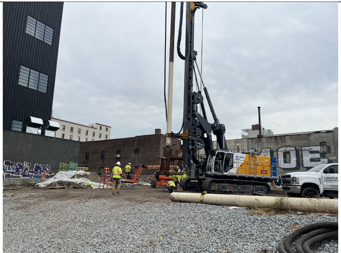
Photo 2- Representative photo of the rod and auger installed on the rig.
