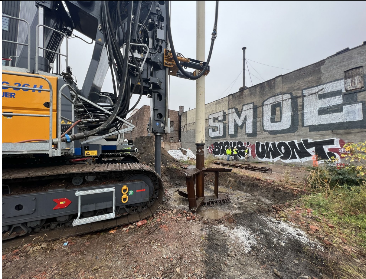
Photo 1- ISS pilot test drilling activities.
