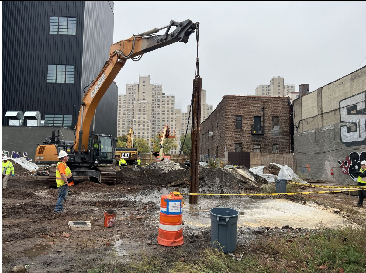
Photo 3- Cascade using sampling rod to collect the QA/QC sample from 30' in column 165.
