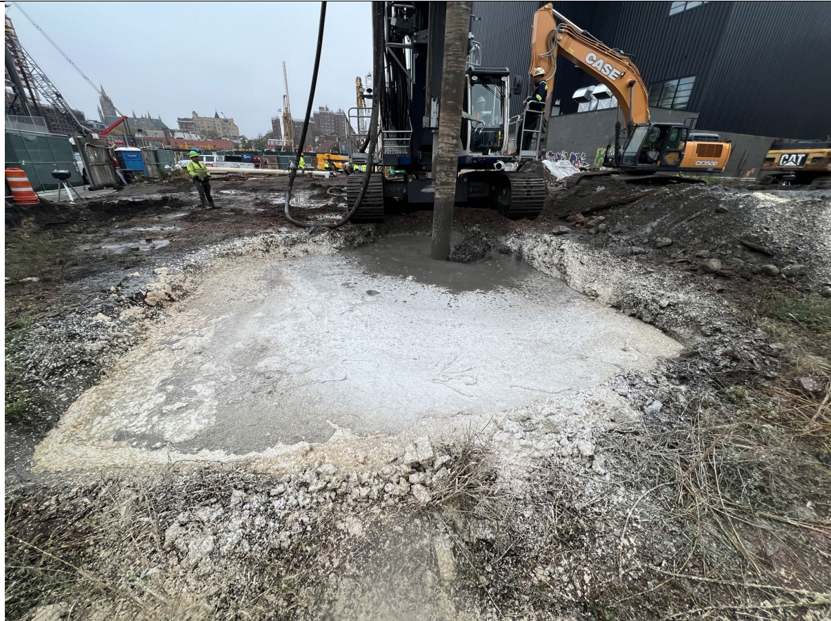
Photo 2- ATMOS foam sprayed to ISS treatment surface to reduce odors.
