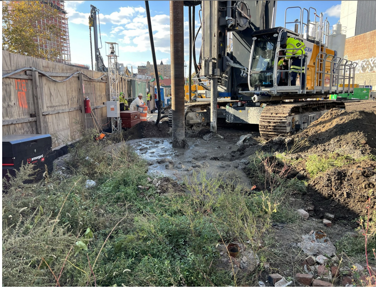
Photo 3- Photo of drilling column 25 with mixture C.
