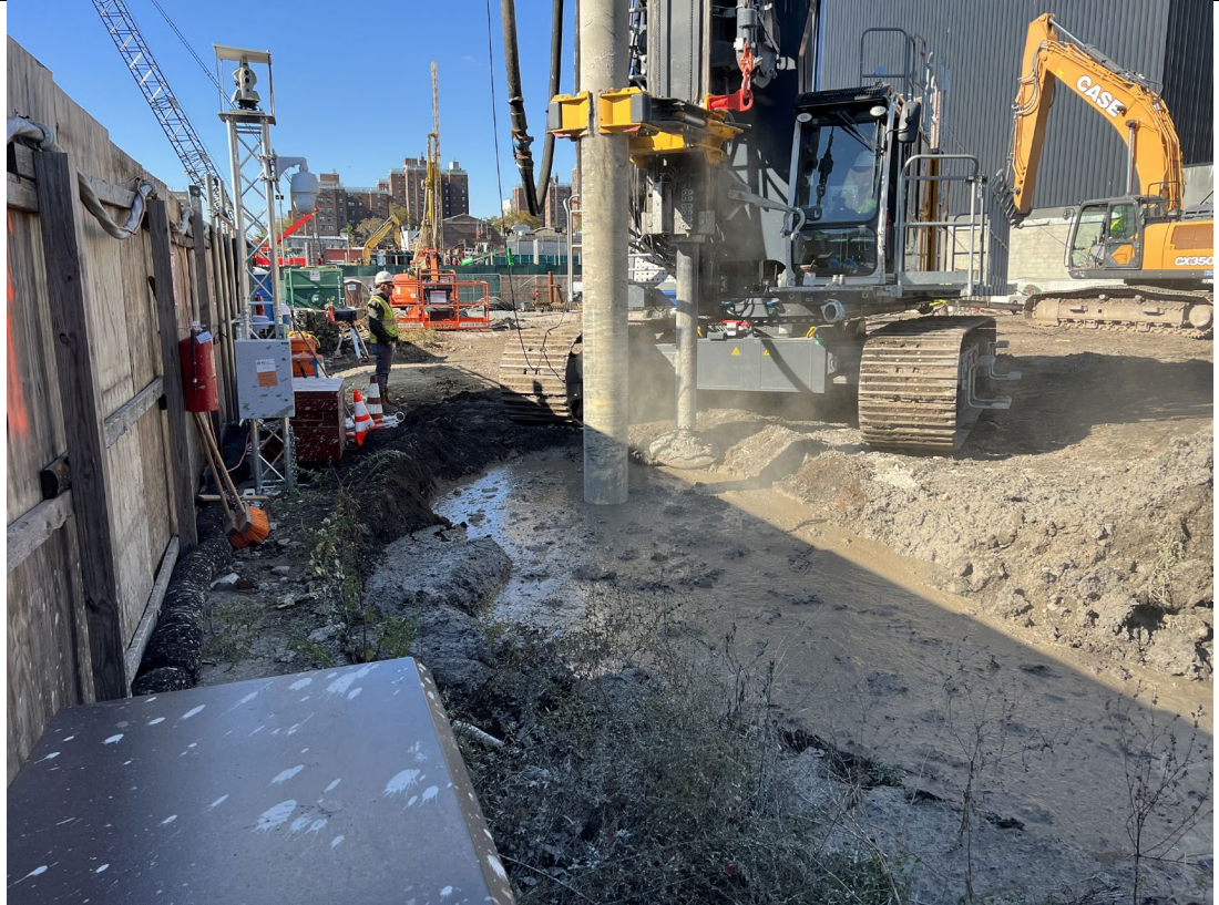
Photo 5- Representative photo of drilling column 24 with mixture C.
