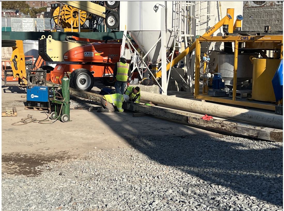
Photo 2- Representative photo of Cascade putting together the additional rod on the sampling tool.
