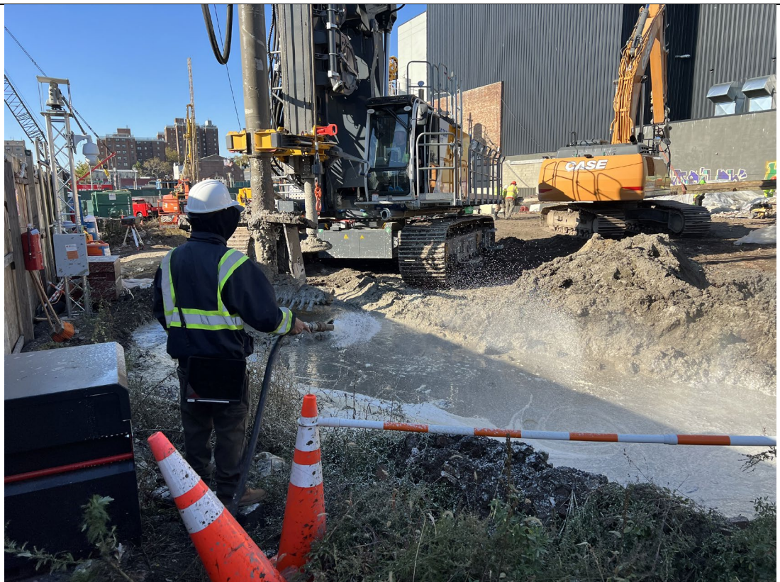
Photo 4- Representative photo of spraying ATMOS foam to mitigate nuisance odors.
