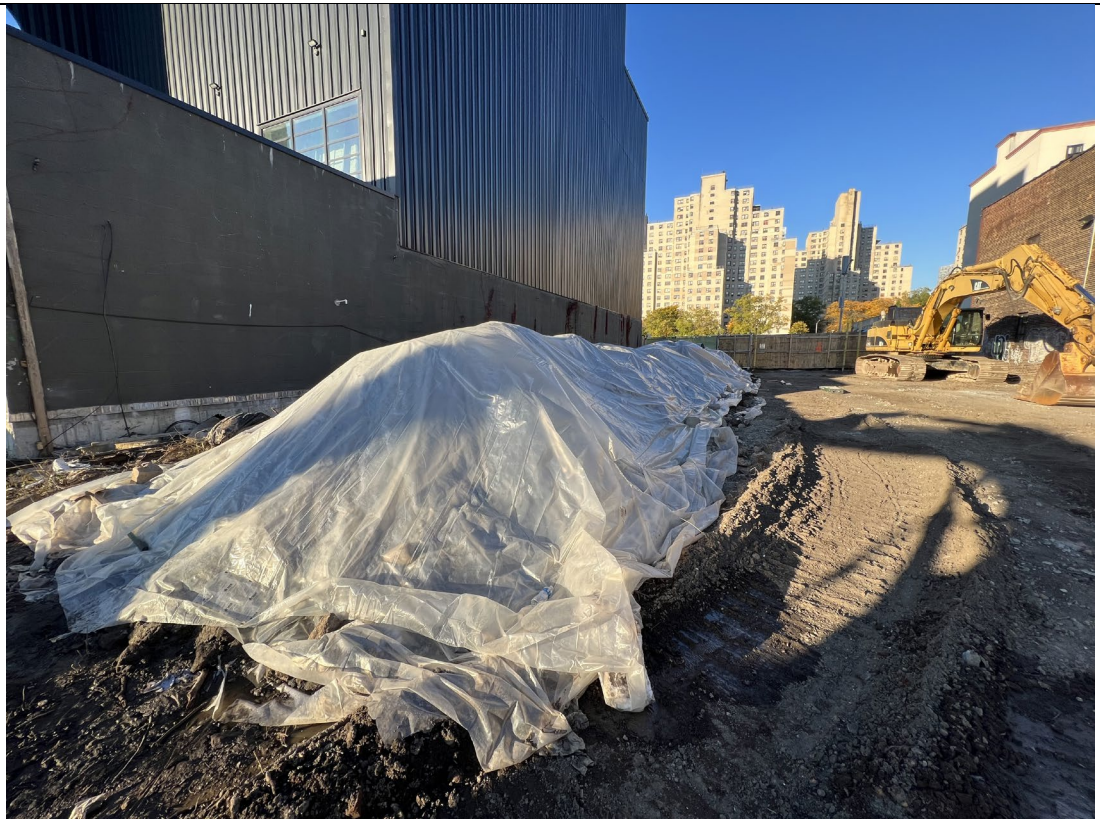
Photo 6- Representative photo of the stockpiled slurry swell covered securely with poly.
