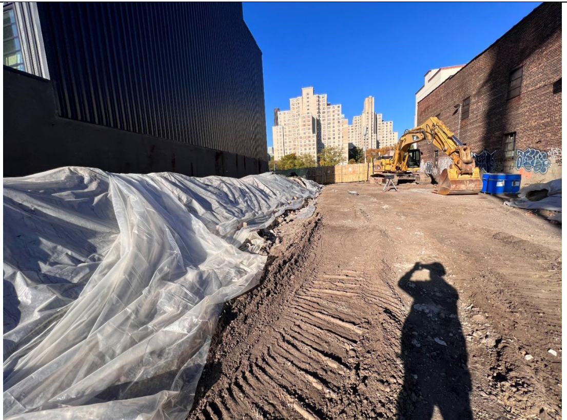
Photo 4- Photo of the stockpiled slurry swell covered securely with poly.
