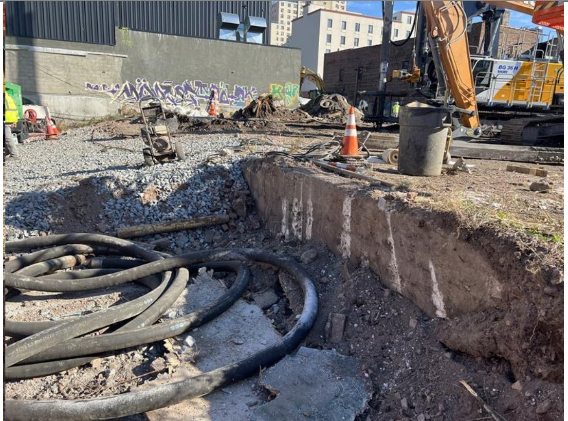
Photo 1- Photo of ramp sideview where treatment columns were proposed.
