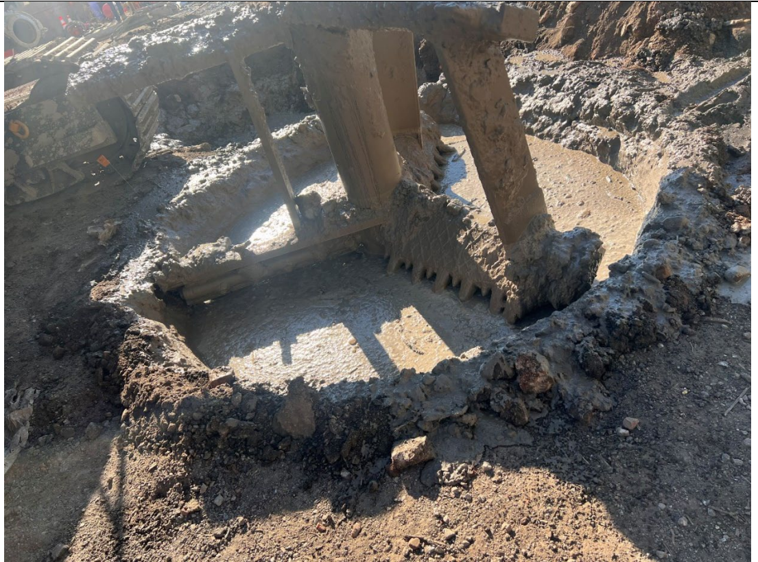
Photo 3- Photo of auger treatment column 304.
